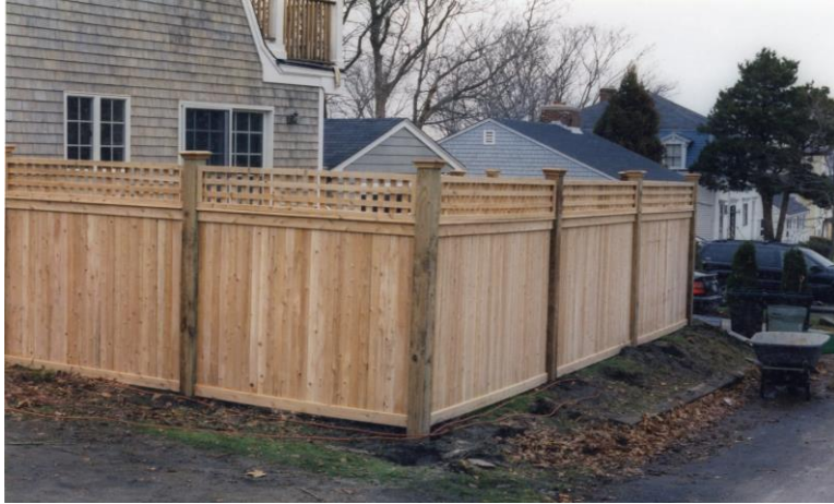
6' high square lattice top fencing with 5x5 posts and post caps
