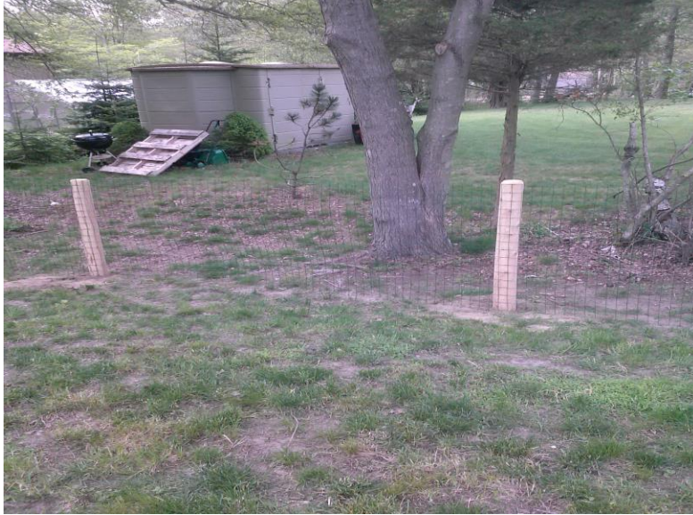
Welded wire attached to round wood posts
