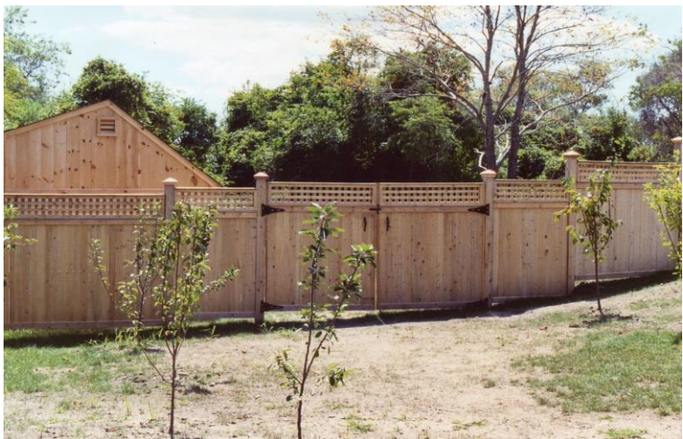
Fence stepping up hill with double gate
