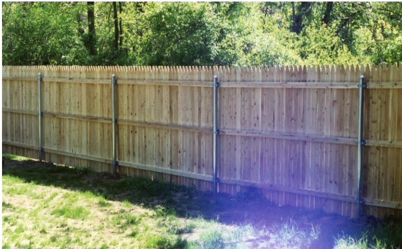
Stockade attached to steel posts
