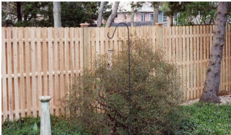
6' high Board on Board style fence dowelled into 5x5 posts
