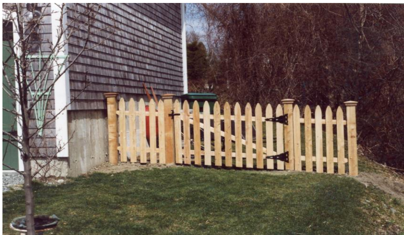
Gothic spaced board fence dowelled into 5x5 cedar posts with caps
