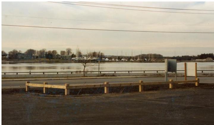
Pressure Treated Guardrail
