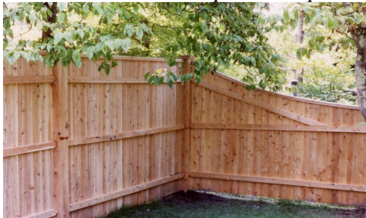
Inside of fence. Fence dowelled into cedar 5x5 posts
