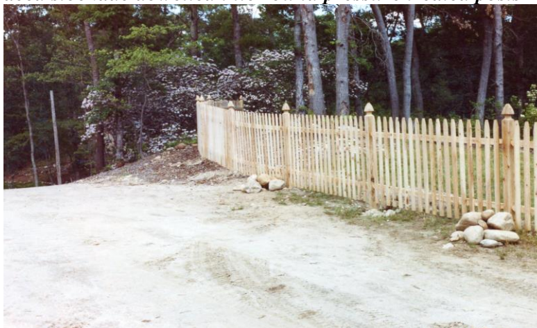
Spaced stockade dowed into 4x4 gothic posts
