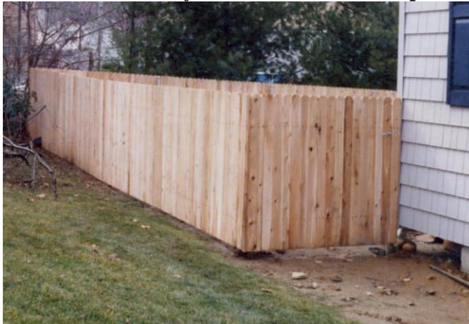
4' high ambassador style fence on steel posts
